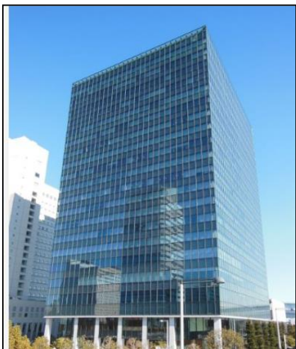
New office located in Ariake Central Tower
